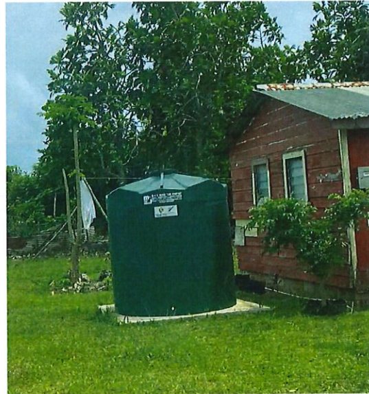
Figure 4: Many households were observed with water tanks installed but no guttering
